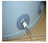
Unscrew the gland nut from the fitting supplied in the tank and also remove locking gland.
