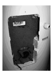
Step 2. Open housing with views of 4 mounting studs
