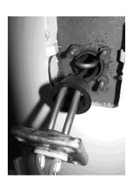
Step 3. Insert element curve facing up & with rubber seal loose on element
