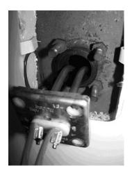
Step 4.Insert rubber seal between element mounting studs.
