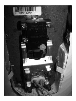
Step 6. Push bracket towards inner tank to tension bracket and clip thermostat under bracket in position.
