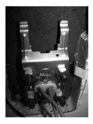
Step 5. Attach thermostat bracket and nuts. Tighten nuts securely & evenly.
