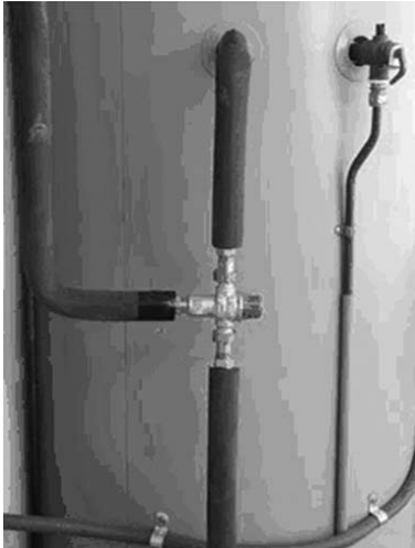
Figure1. A tempering valve attached directly to the cylinder. A second line is required if water in excess of 50 °C is required in the kitchen or laundry.
