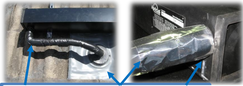
Photo R1 & R2: Roof Connections, all exposed copper is to be insulated without gaps, roof sensor is to be secured to the outside of the insulation (foil tape can be wrapped around pipe and sensor to protect sensor wire) and roof penetration is to be sealed with an approved roof flashing
