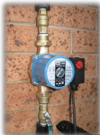
Photo P4: Example of pump location with barrel horizontal, electronics casing positioned on the side with the cable exiting the bottom and solar rated check valve above (required) and ball valve below (recommended)
